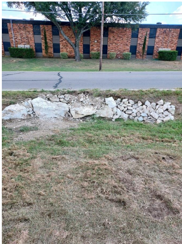
Erosion rock (rip rap) added to wash out areas
