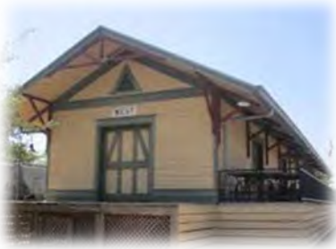
Depot After Restoration
