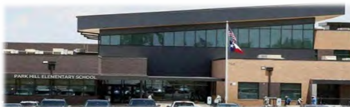
New Park Hill Elementary School built in 2022
