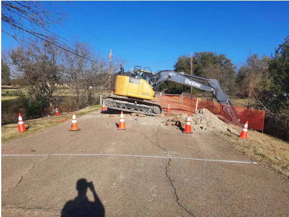
Pipe ditch excavated and on grade
