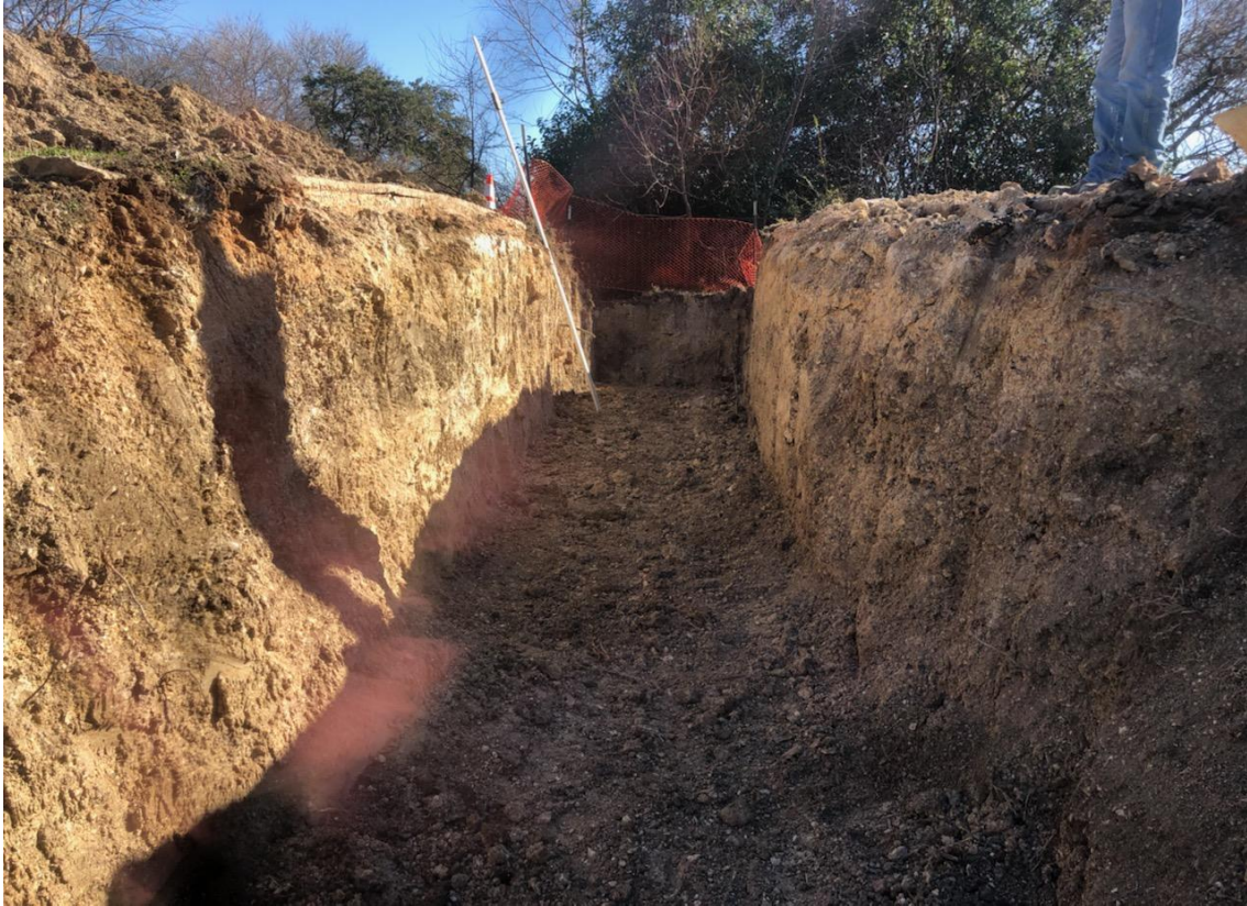
Pipes in place, bedded and backfilled with 1" washrock
