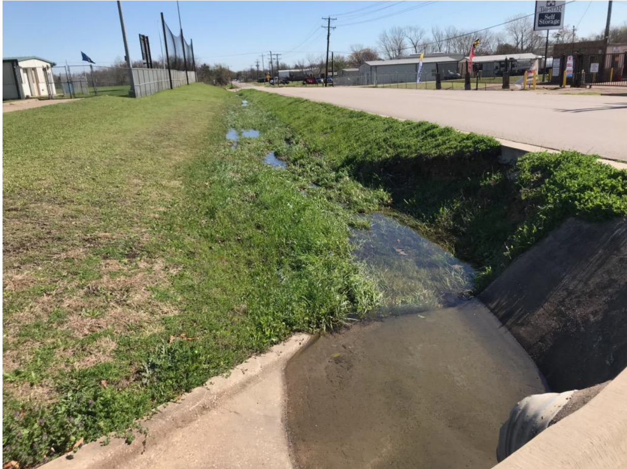
E Panther Way/Fields entrance, erosion of side wall exposing curbing and road base
