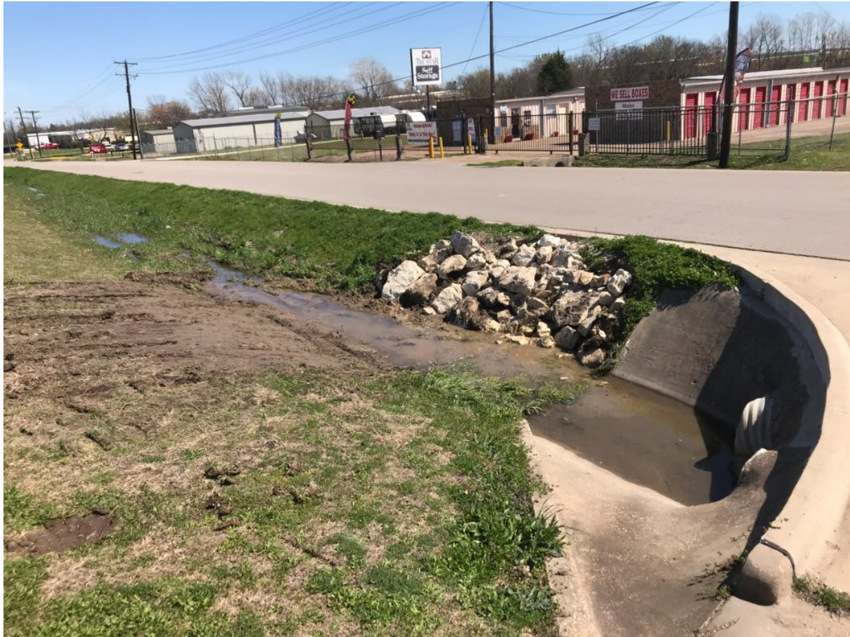
E Panther Way/Fields entrance rip-rap added, silt removed
