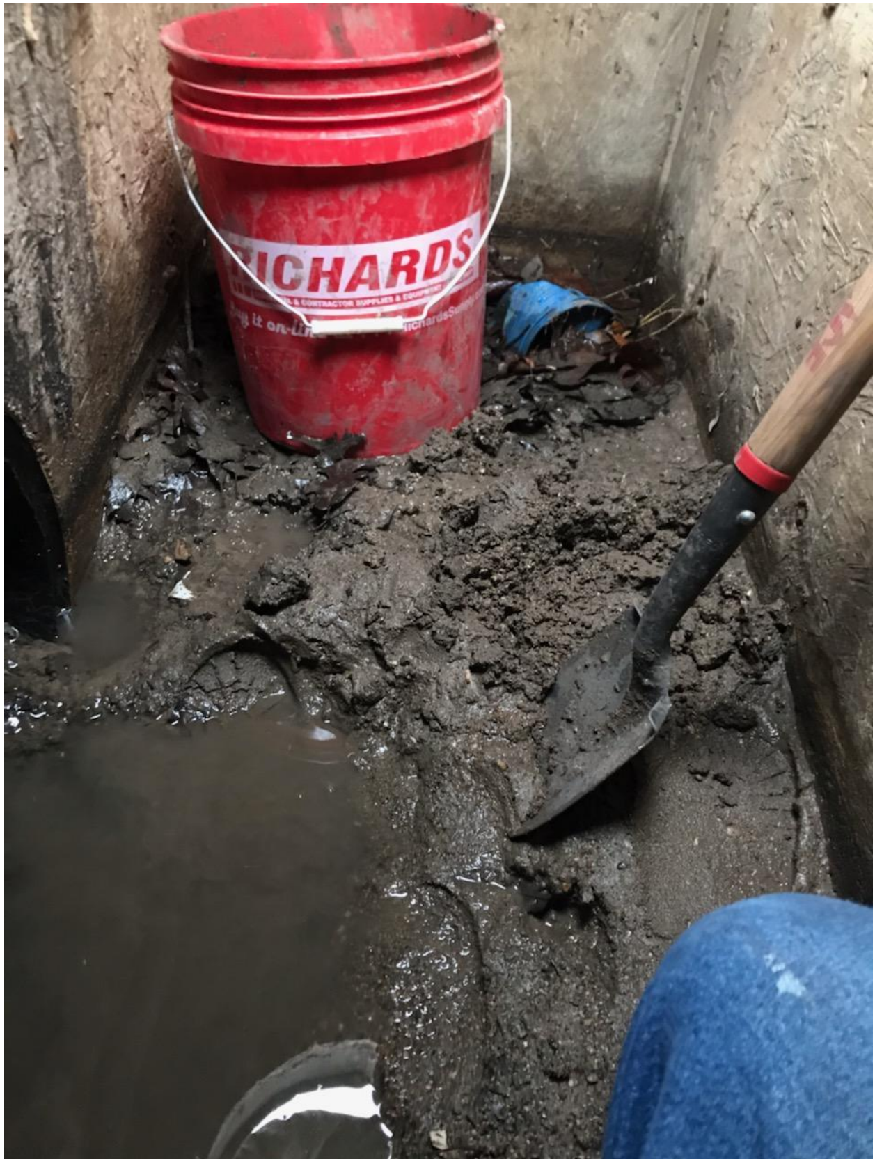
Storm drain box vaults cleaning before/after
